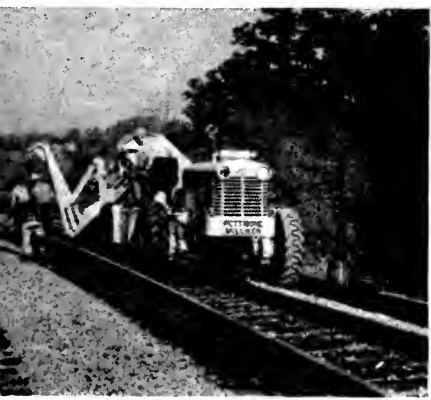
LAYING WELDED RAIL
